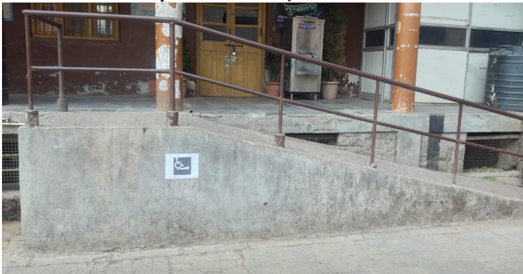
Ramp for the differently abled students
